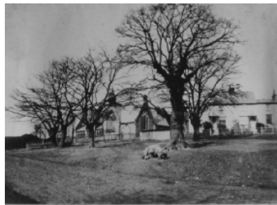
View of the original school c.1890
