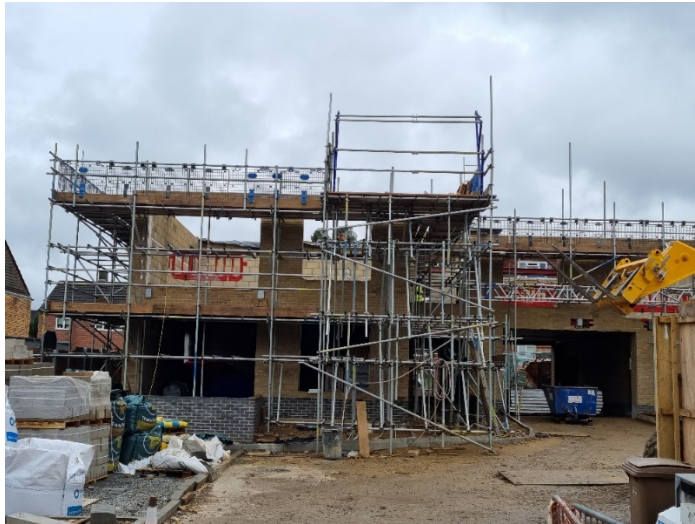
Photo 1 – Construction site at Pentlow Way
