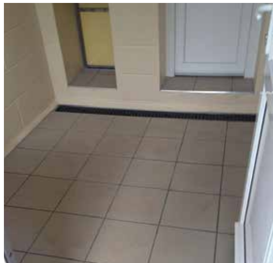
Internal cleanable flooring
