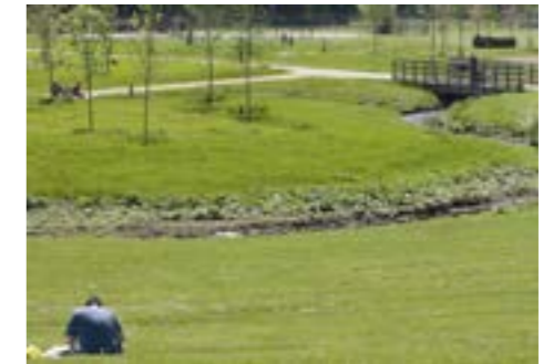
Ladywell Fields, Lewisham (SuDS) Designed to create more sustainable drainage and reduce flooding, the river channel was modified to create a naturalistic setting incorporating backwaters and wetlands.
