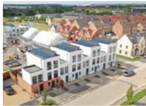
Project Etopia, Corby Uses combined solar PV's and thermal panel to deliver net zero carbon on site.
