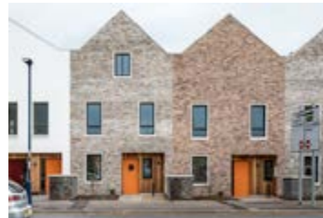
Marmalade Lane, Cambridge Built with fabric-first approach for energy efficient homes, alleviating fuel-poverty.
