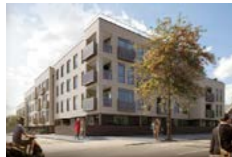
Tallack Road, Waltham Forest, London Large-scale communal Air Source Heat Pump to feed ambient temperature heat network
